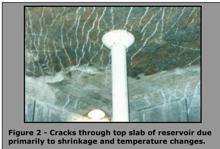
**Figure 2 - Cracks through top slab of reservoir due primarily to shrinkage and temperature changes.**
