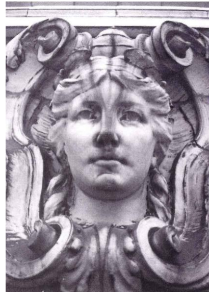
Close up of typical terra cotta work found on many Chicago area properties.
